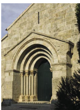
6. West façade. The portal is inserted in a stone structure stemming from the façade to appear deeper, a solution similar to the portals of the churches of the Savior of Unhão (Felgueiras), Saint Vincent of Sousa (Felgueiras) and Saint Peter of Ferreira (Paços de Ferreira).
