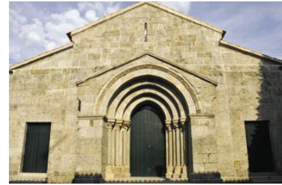
2. Although the church is composed of three naves, planimetrics corresponding to an enlargement made in the Modern Period, the Romanesque construction featured a single nave.
