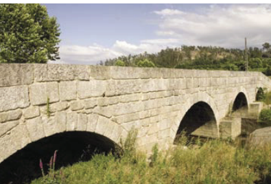
3. To the river basin, Vilela Bridge's cut-waters are quadrangular.
