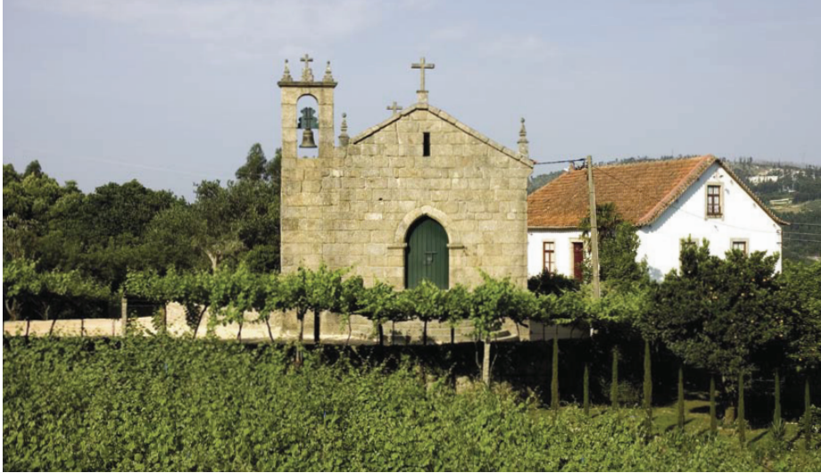
2. West façade. Even though early mentions to it are traced back to the 11th century, this church's present state corresponds to a restoration not prior to the 14th century.
