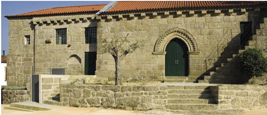
5. South façade. This façade's portal presents the same decorative solution as the triumph arch inside the church. The transept was lengthened and heightened after the original construction.
