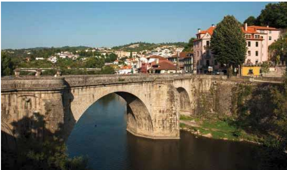
Bridge of Saint Gonçalo (Amarante). Downstream view.
