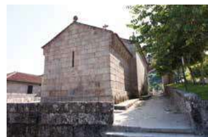
East and north façades.
