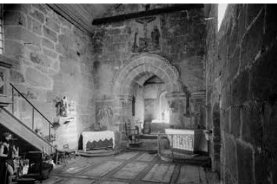
Nave before the intervention carried out by the DGEMN. Source: IHRU archive.
