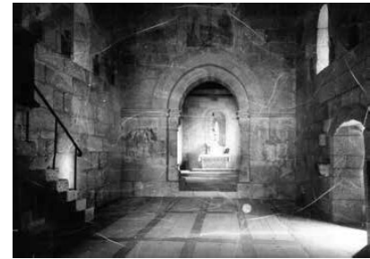
Nave after the intervention carried out by the DGEMN. Source: IHRU archive.
