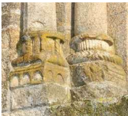
North façade. Nave. Portal. Bases.
