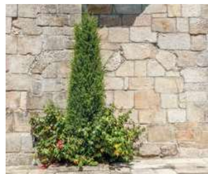
South façade. Nave. Traces of arches.
