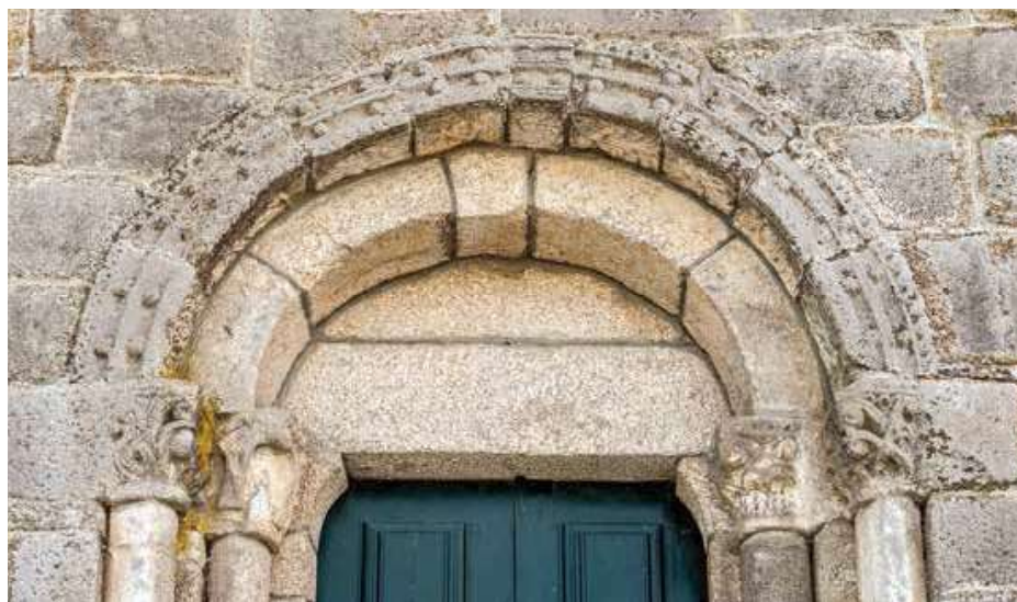
North façade. Nave. Portal. Tympanum, archivolts and capitals.
