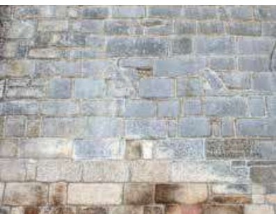
North façade. Nave. Wall.
