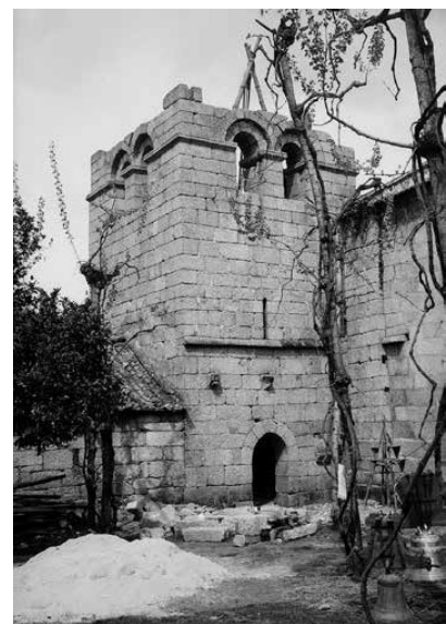
Church. Demolition works of the high choir. Source: IHRU archive.
