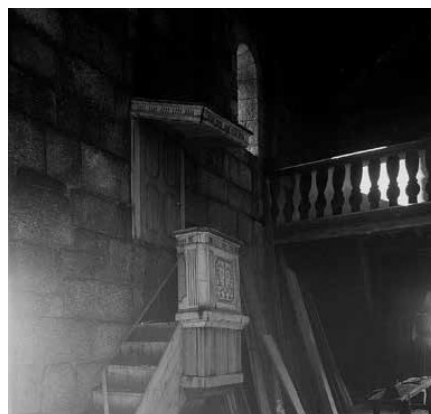
Church. Demolition works of the high choir. Source: IHRU archive.
