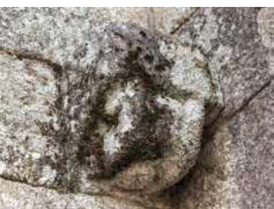
Bell tower. East façade. Carved ashlar.
