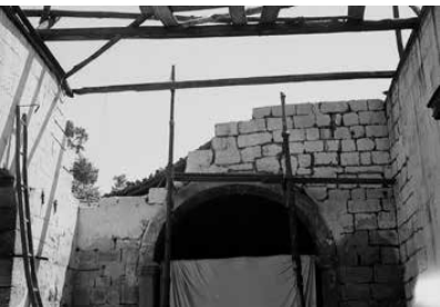
Demolition and reconstruction works of the triumphal arch's gable and part of the north wall. Source: IHRU archive.
