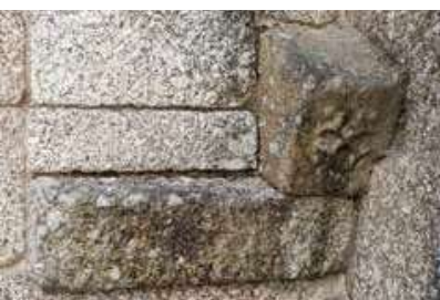
Bell tower. East façade. Carved ashlar.
