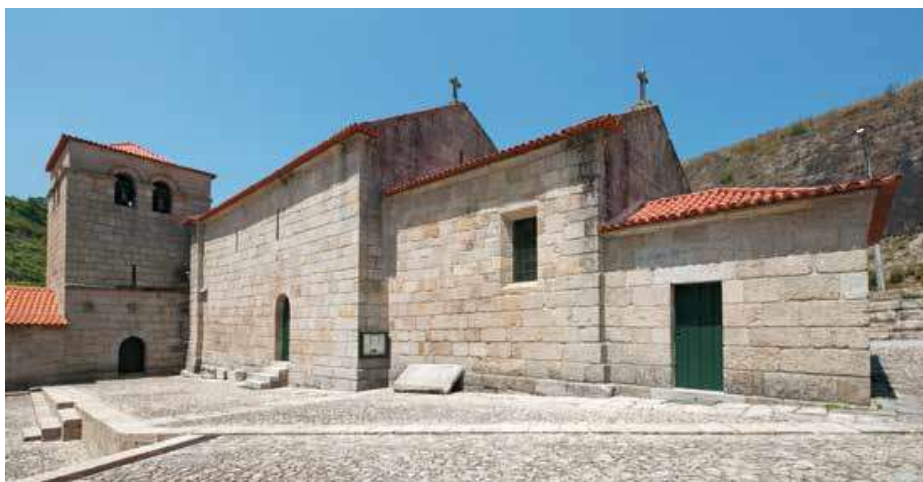
Church. South façade.
