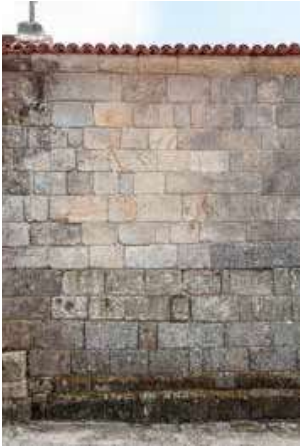
Church. North façade. Chancel. Scars detail.
