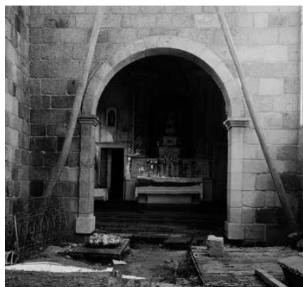
Church. Removal works of the interior plaster. Source: IHRU archive.
