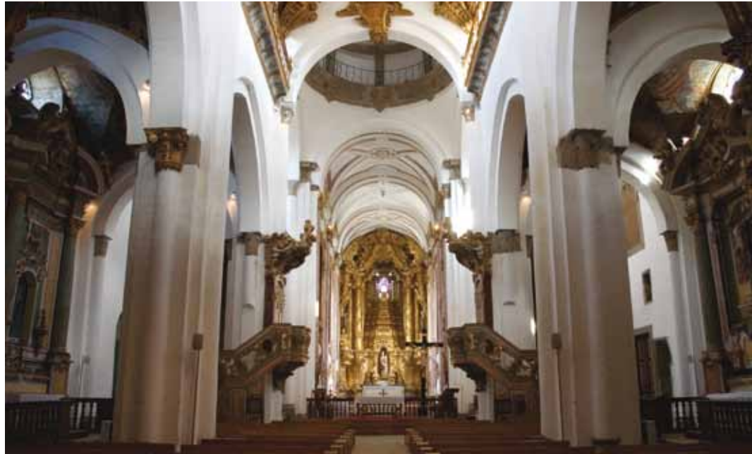
10. Composed of three naves, the church of Saint Mary of Pombeiro features a system of diaphragms arches matching the same typology as that of the monastic church of Paço de Sousa. The decoration from the Baroque period has not altered the naves' structure.
