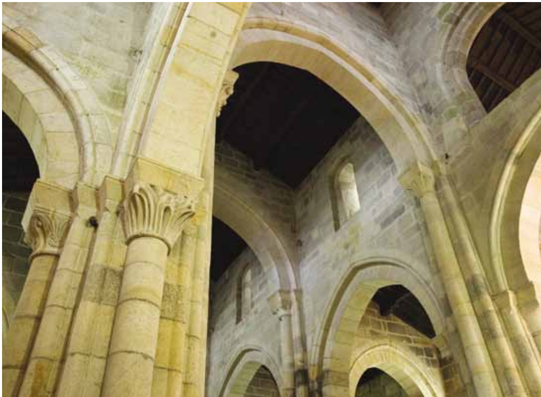
11. Transept roofing of the central and lateral naves. The diaphragm arches alternate with wood cover.
