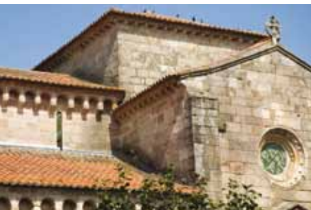
14. The transept's upper portion and the tower over the cross correspond to the last construction stage.
