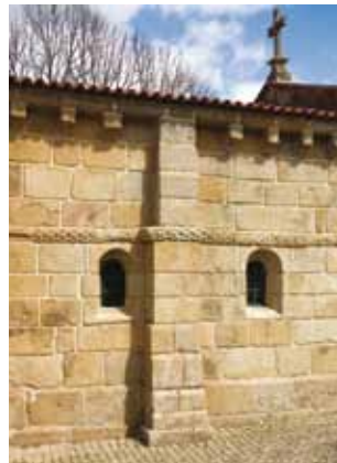
4. The step buttresses are meant to minimize the infiltration of rain water inside the walls. The sculpted frieze resumes themes of Hispanic-Visigothic tradition, in a solution that is very common in the Sousa Valley's Romanesque.
