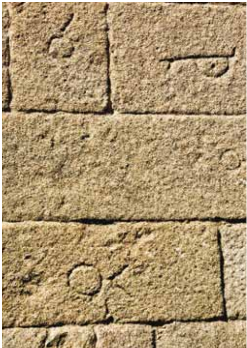
4. Alphabetical and geometrical signs. These masonry markings were used to account for the mason's work. Boelhe's signs, frequent and repeated, suggest that the church was probably made by half a dozen masons.
