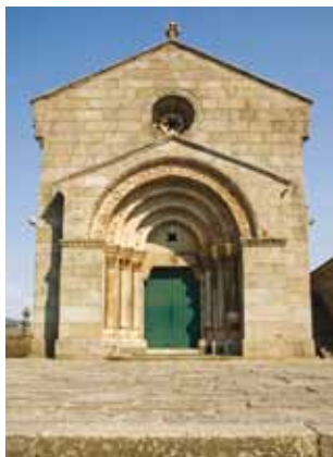
4. West façade. The portal is inserted in a pentagonal structure stemming from the façade, a usual solution in this region, as the church portals of Saint Mary of Airões and of the Savior of Unhão, both in the municipality of Felgueiras, demonstrate.
