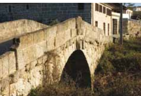
4. At Espindo bridge, the span has forced the elevation of the arch and the positioning of the tray in trestle.
