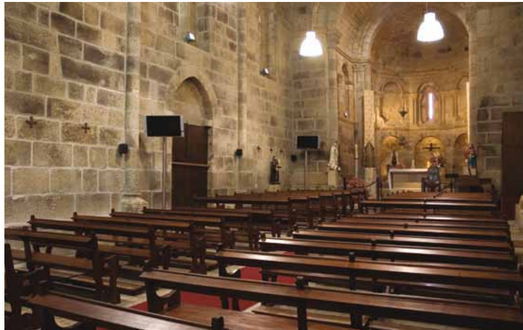
12. The church nave has received columns adjacent to the walls. The reason for the existence of columns, corresponding to buttresses on the exterior, is related to the nave's great height.
