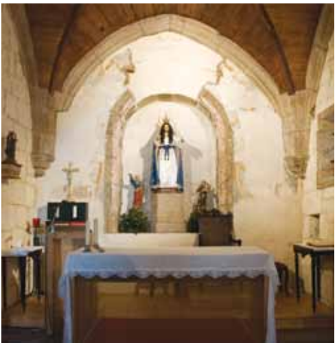
3. Transept. The corbels and the Manueline framework point to a construction, or reconstruction, traceable to the late 15 th or early 16 th century.
