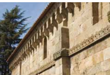
15. South façade. In the cornice, the arches of the lateral nave are supported by corbels. The frieze stretching along the wall, in Pre-Romanesque architecture fashion, is one of the most characteristic aspects of this church.
