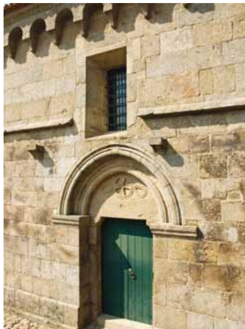
7. South façade. The drip course and corbels testify to the presence of a one story high porch or a cloister.
