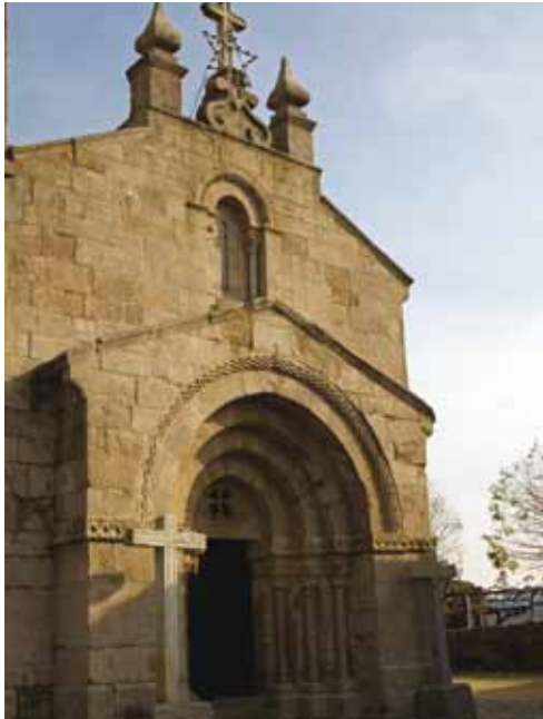
6. West façade. The portal, encased in a stone structure, has a construction projection similar to that of the church façades of Saint Vincent of Sousa and Saint Mary of Airões, also in the municipality of Felgueiras.
