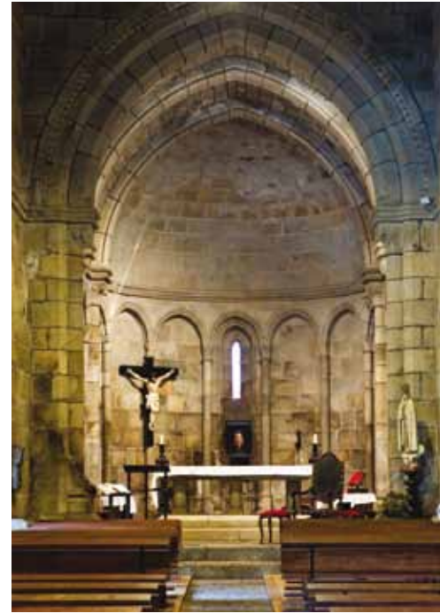
10. The transept shows blind arcades livening up the wall surface. This solution, common in Romanesque architecture, is also used during the Gothic period.
