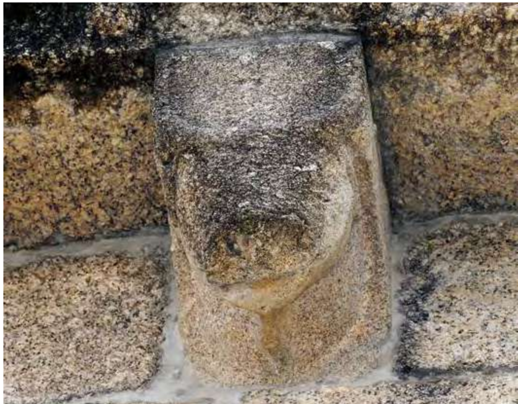
North wall. Nave. Corbel.
