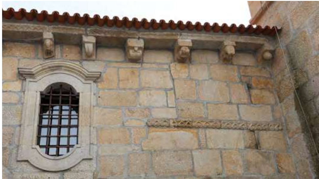
North façade. Nave. Frieze and later works.
