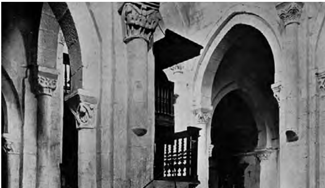
Church. Interior view before the intervention carried out by the DGEMN. Source: DGEMN's Bulletin no. 15.
