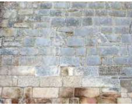
North façade. Nave. Wall.
