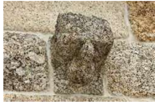
South façade. Nave. Corbel.
