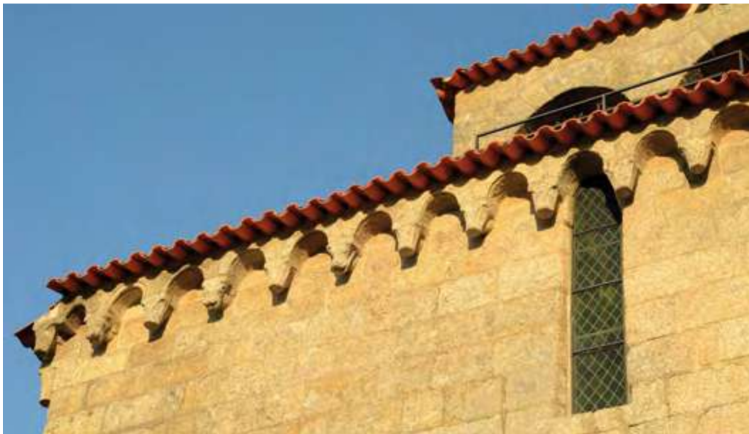
West façade. Corbels.
