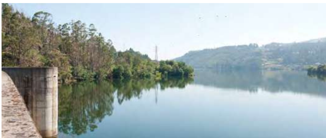
Torrão dam. View of the reservoir.
