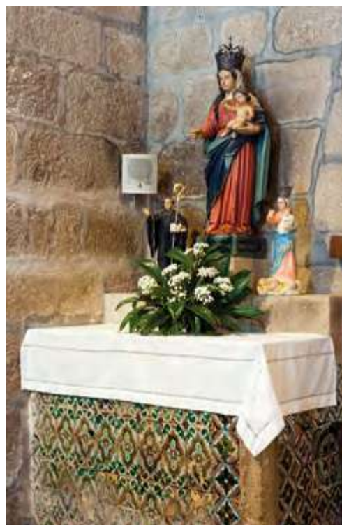
Triumphal arch. Wall on the Gospel side. Collateral altarpiece after the intervention carried out by the DGEMN.
