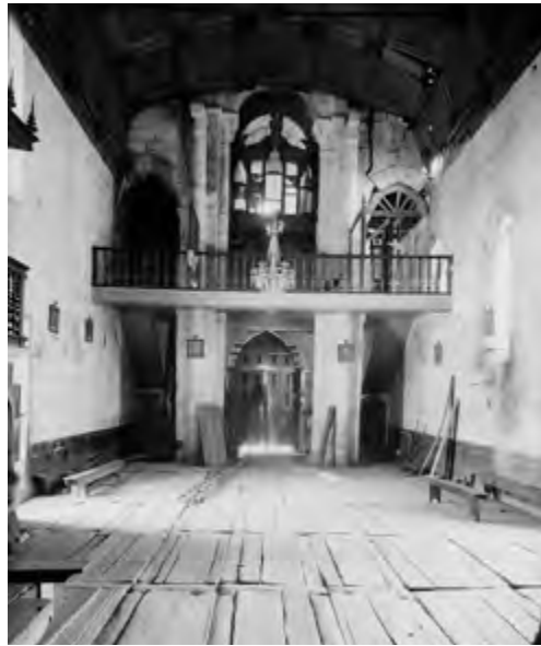
Nave before the intervention carried out by the DGEMN. Source: IHRU archive.
