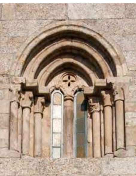
West façade. Mullioned window.
