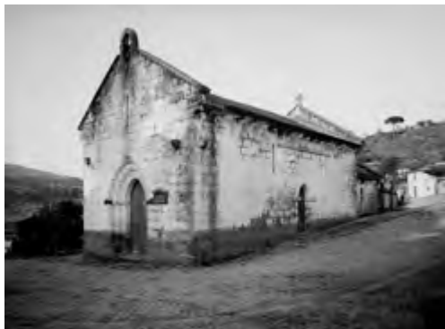
West and south façades before the intervention carried out by the DGEMN (1944). Source: IHRU archive.
