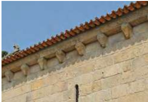
South façade. Nave. Corbels.
