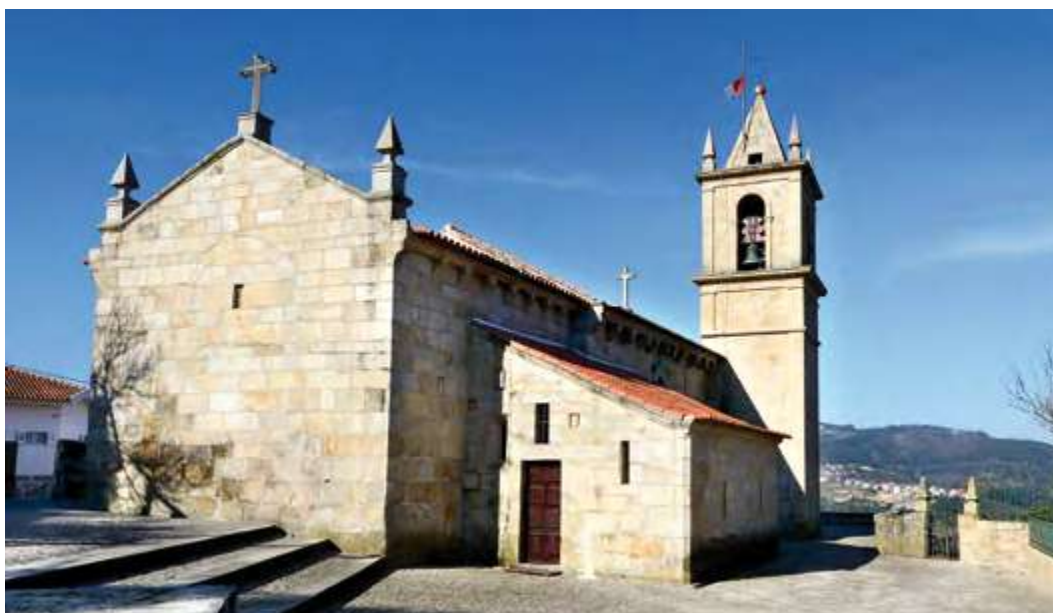
East and north façades.
