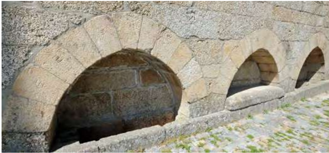
South façade. Nave. Arcosolia.
