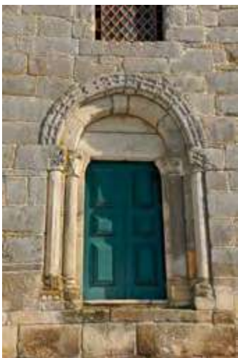
North façade. Nave. Portal.
