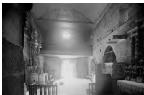
Nave before the intervention carried out by the DGEMN. Source: IHRU archive.
