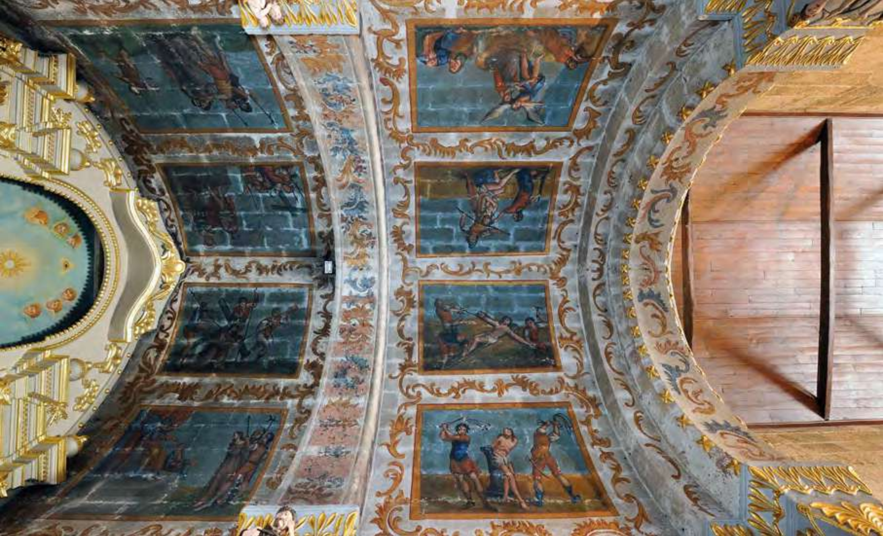
Chancel. Vault. Paintings.
