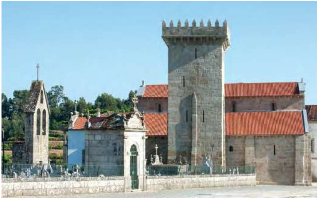
Church and tower. North façade.
