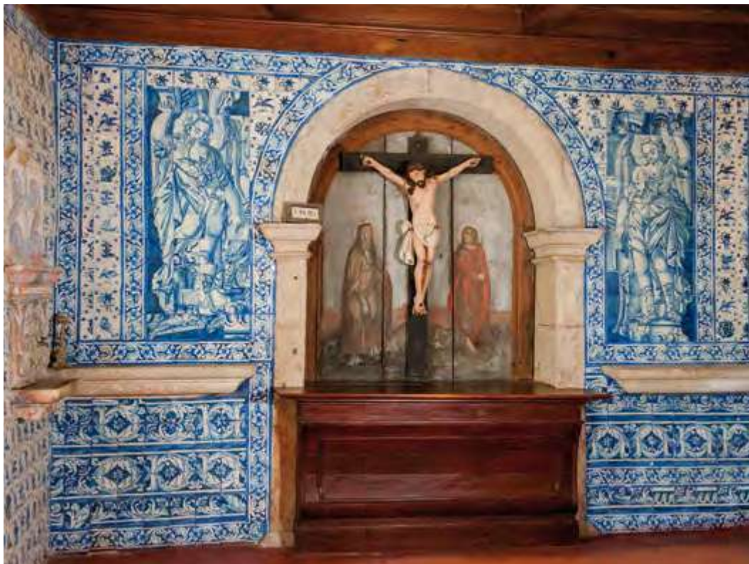
Sacristy. Tile lining, washbasin and altarpiece.
