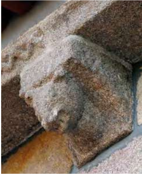
South façade. Nave. Corbel.
