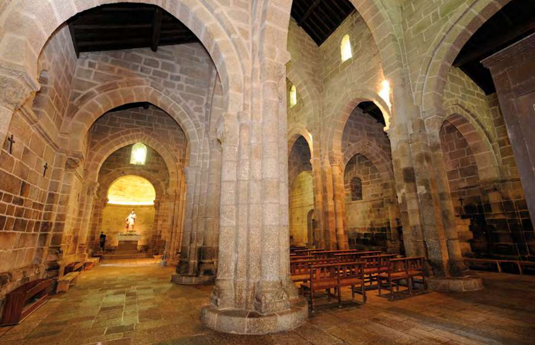
Church. Naves. Diaphragm arches.
