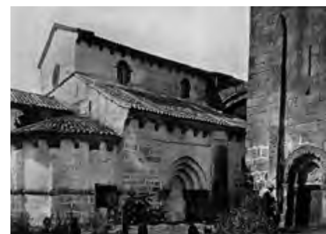
Church. Chancel and apse before the intervention carried out by the DGEMN. Source: DGEMN’s Bulletin no. 15.
