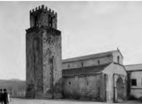
Church and tower before the intervention carried out by the DGEMN. Source: IHRU archive.
