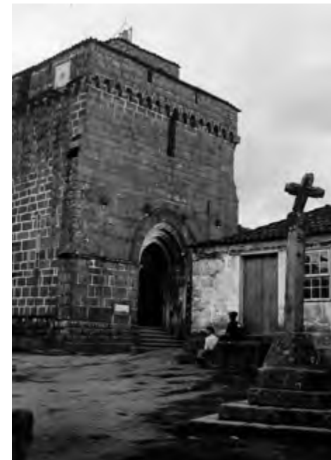
West façade and churchyard before the intervention carried out by the DGEMN. Source: Nuno Resende's private collection.
