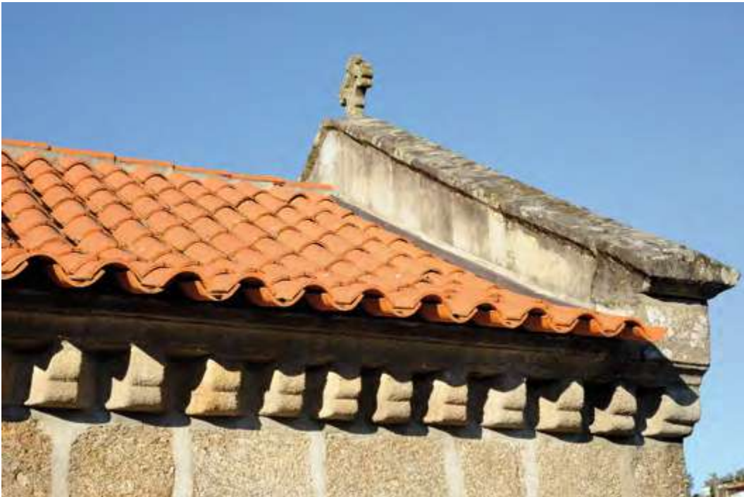
South façade. Chancel. Corbels.
