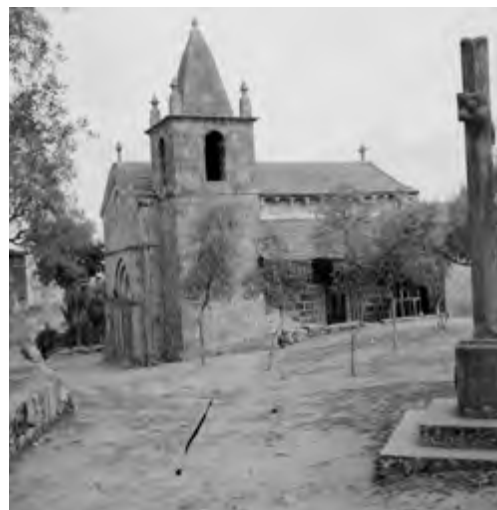
General external view before the intervention carried out by the DGEMN (1960). Source: IHRU archive.
