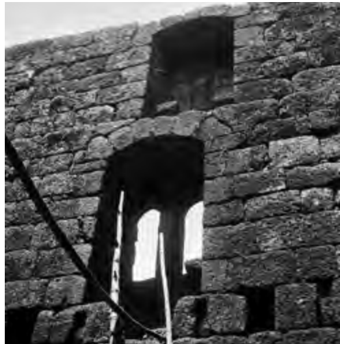
Northeast façade. Intermediate floor. Detail of the mullioned window (interior view) (1951). Source: IHRU archive.
