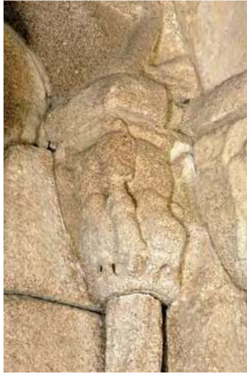
Chapel of Saint John the Baptist. Crevice. Capital.
