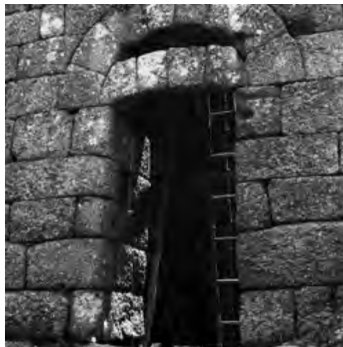
Northeast façade. Door (1951). Source: IHRU archive.
