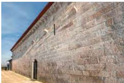
North façade. Nave.
