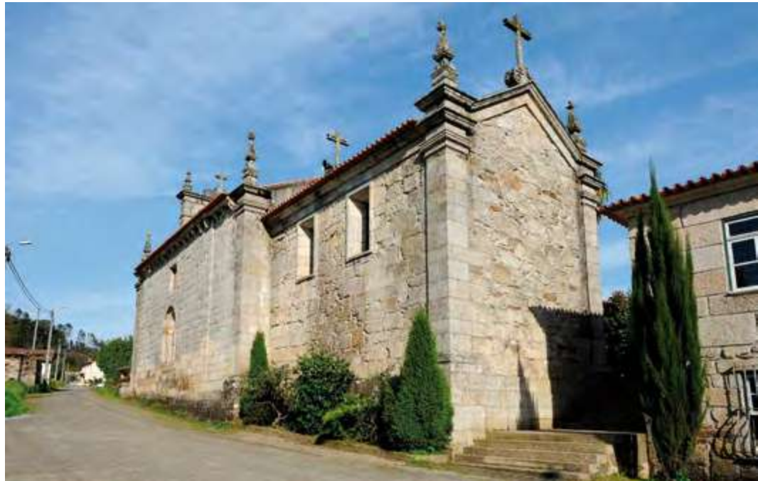
North and west façades.
