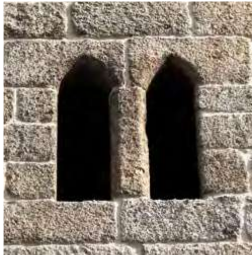
Northeast façade. Upper floor. Detail of the mullioned window. External view.
