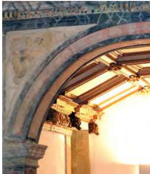
Church. Arch that supports the choir. Painting detail.
