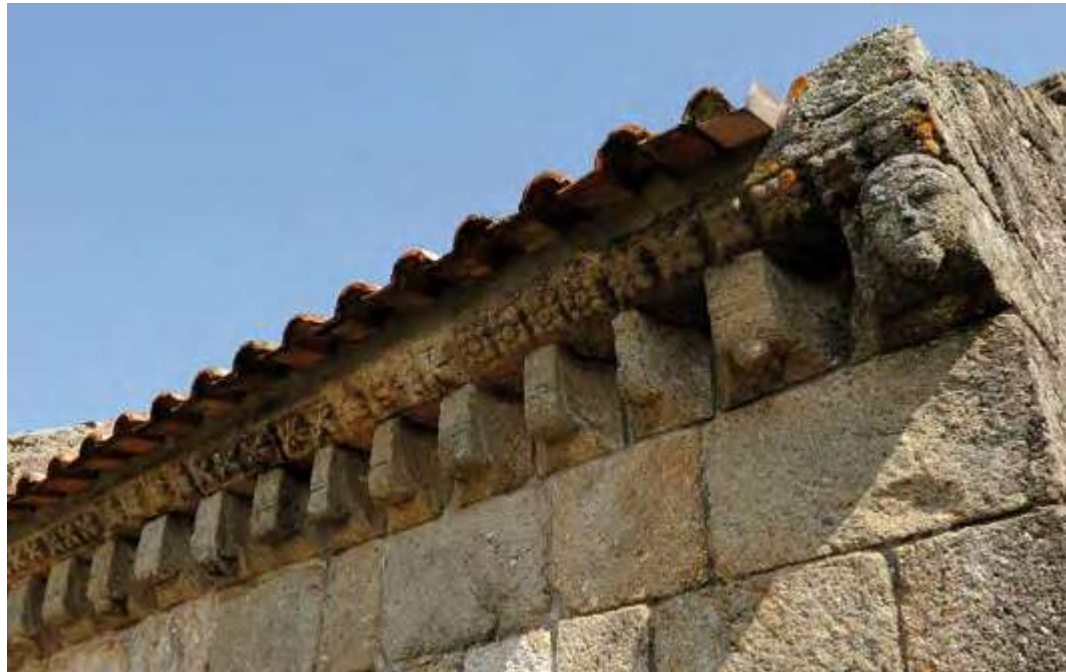
South façade. Chancel. Corbels.
