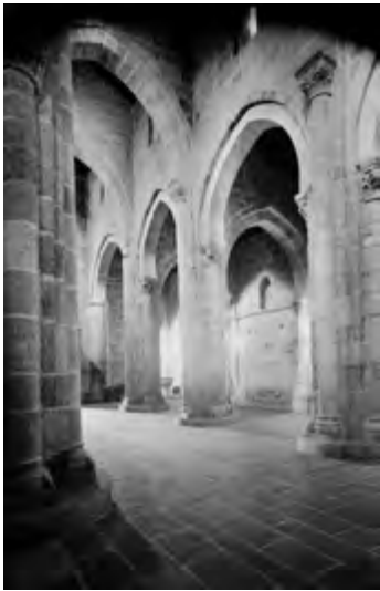
Church. Interior view after the intervention carried out by the DGEMN. Source: IHRU archive.
