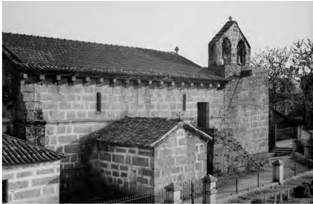
North façade before the intervention carried out by the DGEMN. Source: IHRU archive.
