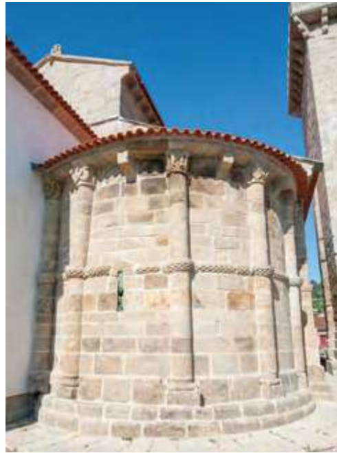
Church. North apse chapel.
