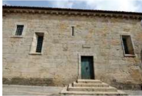
South façade. Nave.
