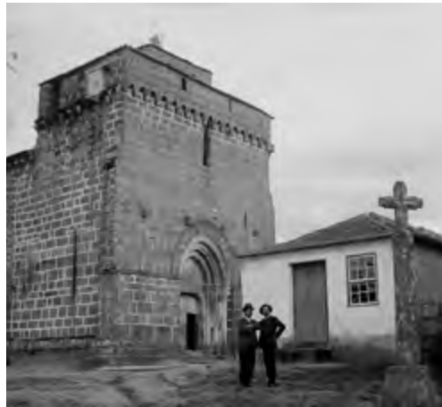
West façade and churchyard before the intervention carried out by the DGEMN. Source: IHRU archive.
