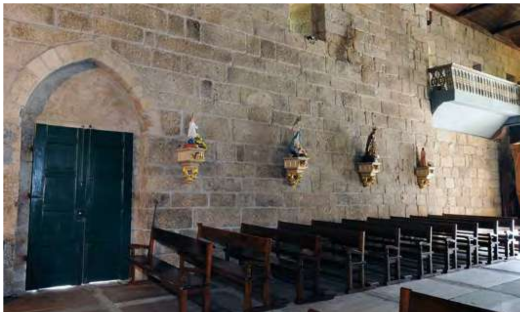
Nave. South wall.
