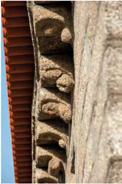
North façade. Nave. Corbels.
