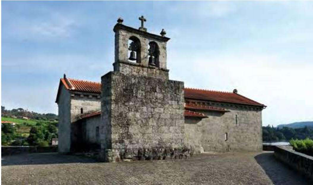
Church of Sobretâmega. North façade and bell tower.
