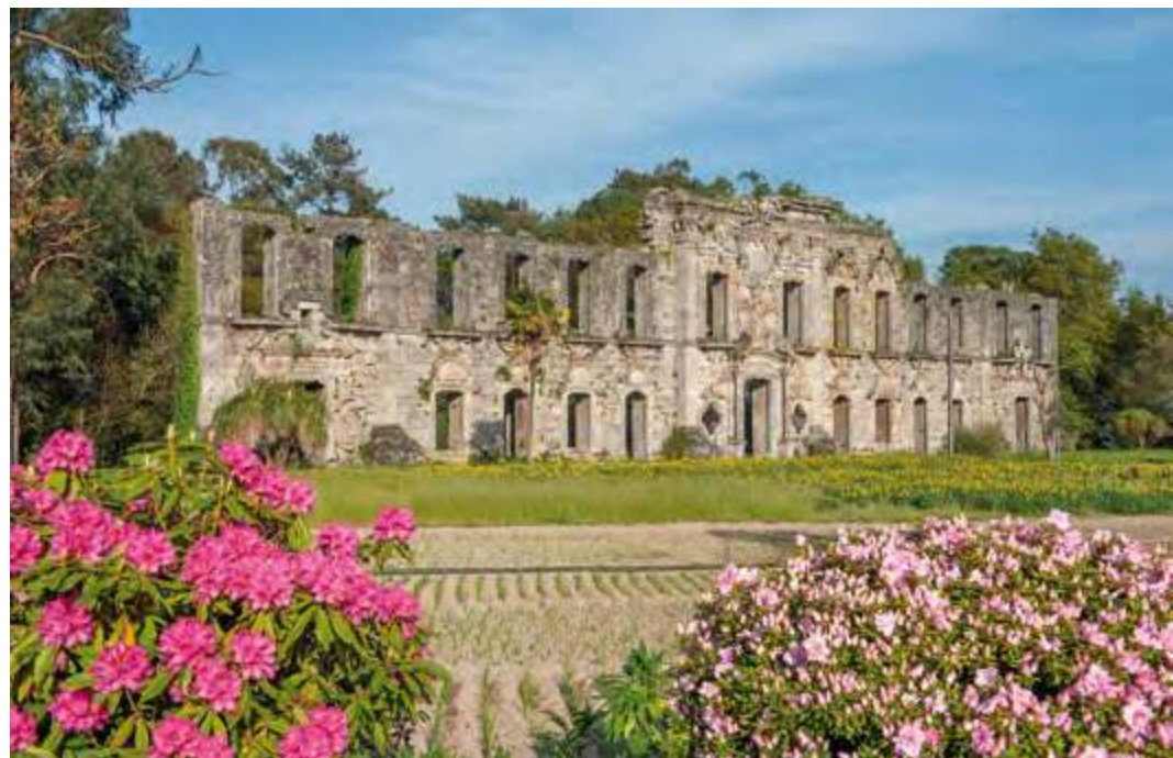
Façade of the (unfinished) noble house of the Portocarreiros (also known as the unfinished palace of Vila Boa de Quires or the fidalgo's works) (Marco de Canaveses).
