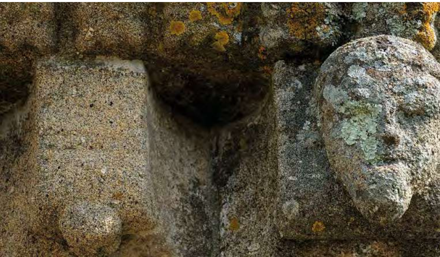
South façade. Chancel. Corbels.
