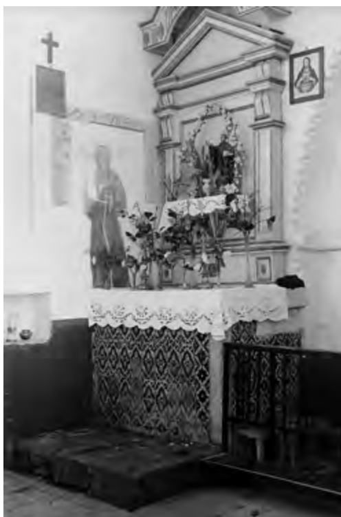
Triumphal arch. Wall on the Gospel side. Collateral altarpiece before the intervention carried out by the DGEMN (1944). Source: IHRU archive. It is possible to see in the image a mural painting that no longer exists.
