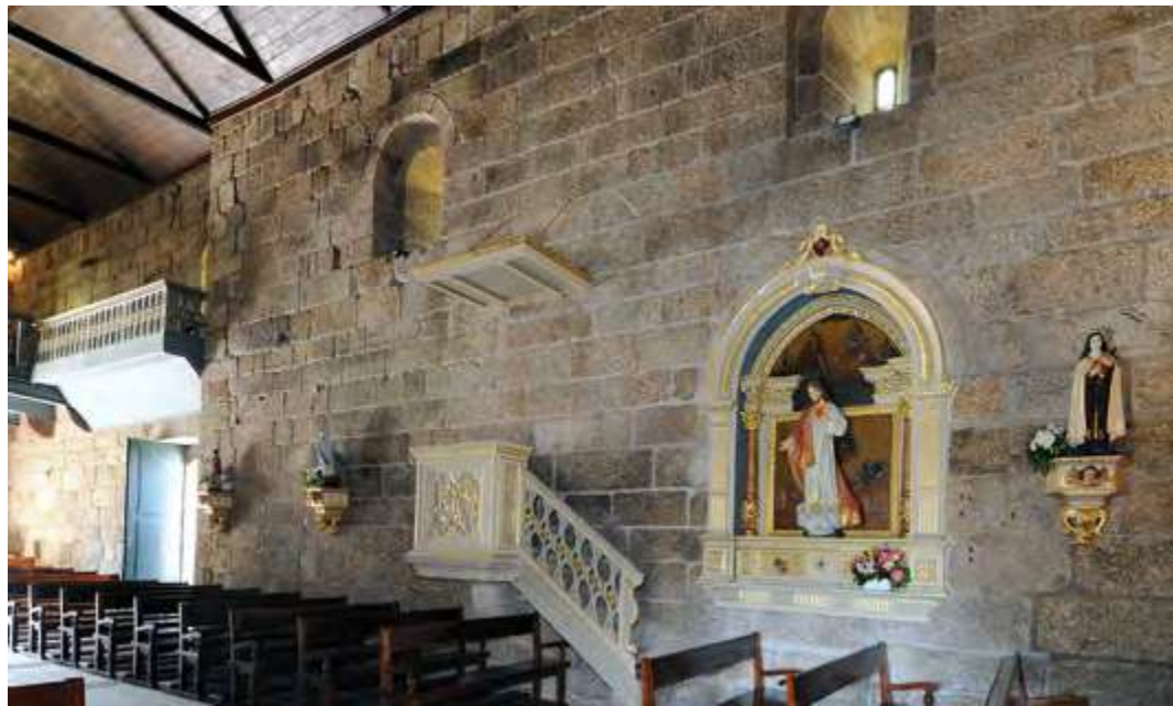
Nave. North wall.
