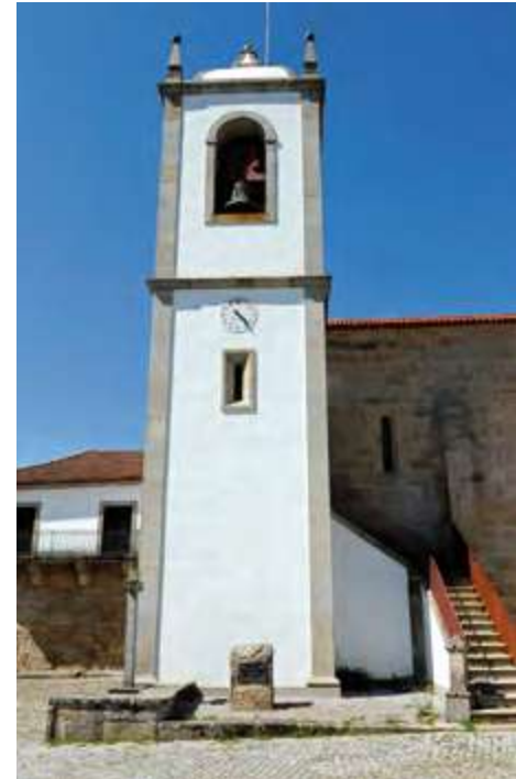
South façade. Bell tower.
