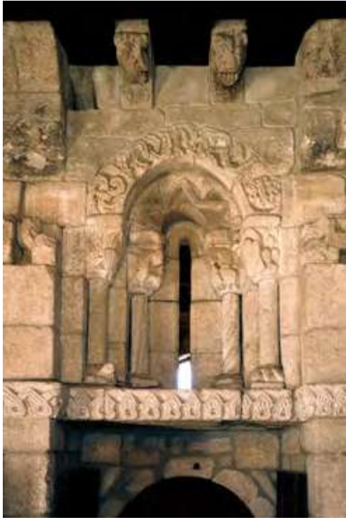
Chapel of Saint John the Baptist. Crevice.
