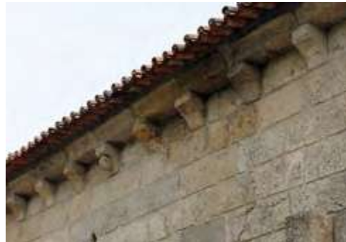
North façade. Nave. Corbels.
