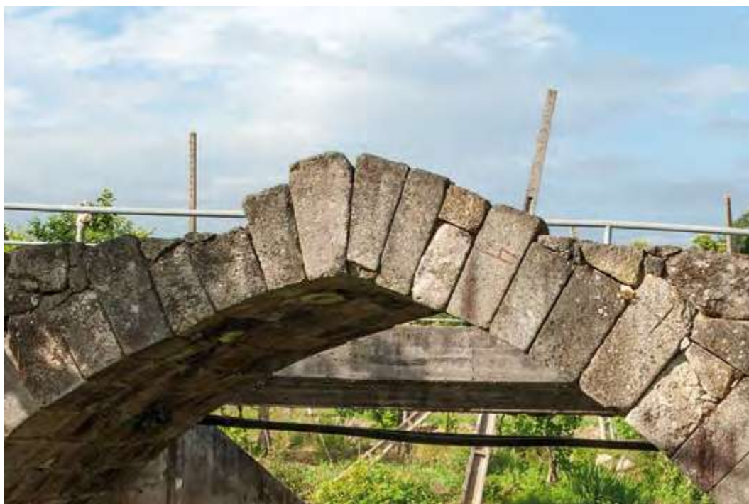
Downstream view. Arch top.
