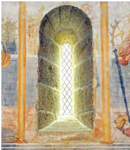
Chancel. Back wall. Crevice.
