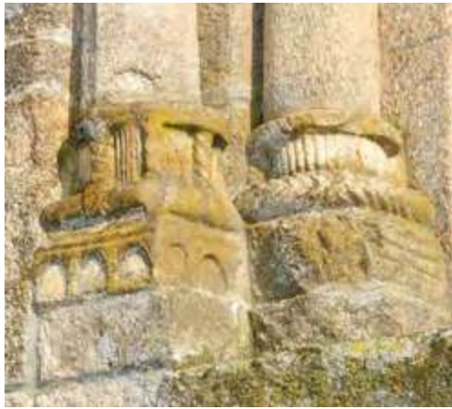
North façade. Nave. Portal. Bases.
