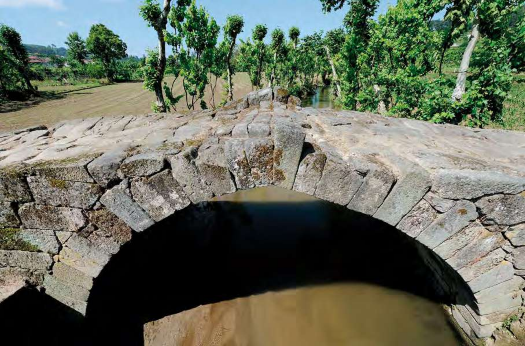
Upstream view. Arch and platform.
