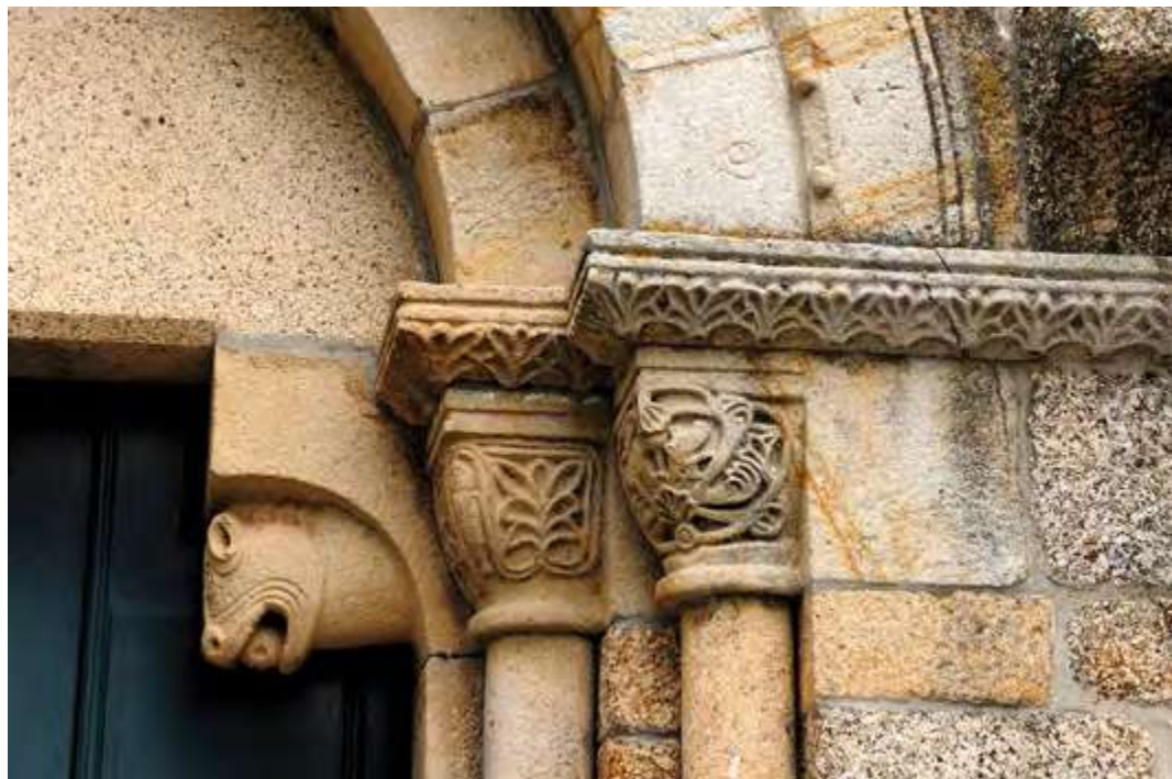
South façade. Nave. Portal. Corbel, capitals and imposts.
