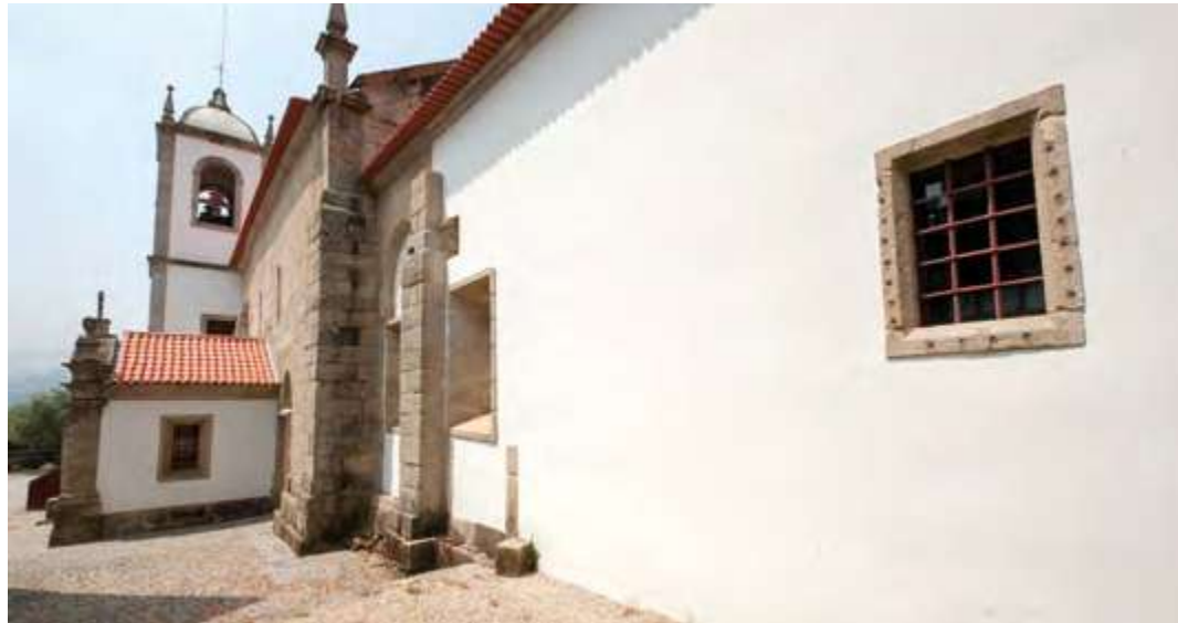
Church. South façade.
