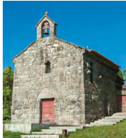
Church of Vila Verde (Felgueiras). West and south façades.
