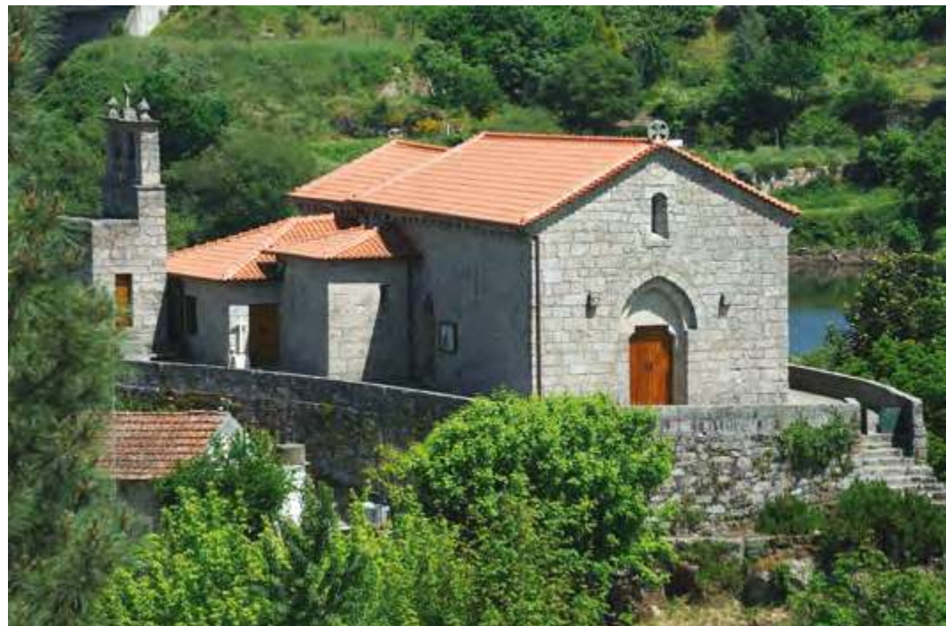
Church of Sobretâmega. General view.
