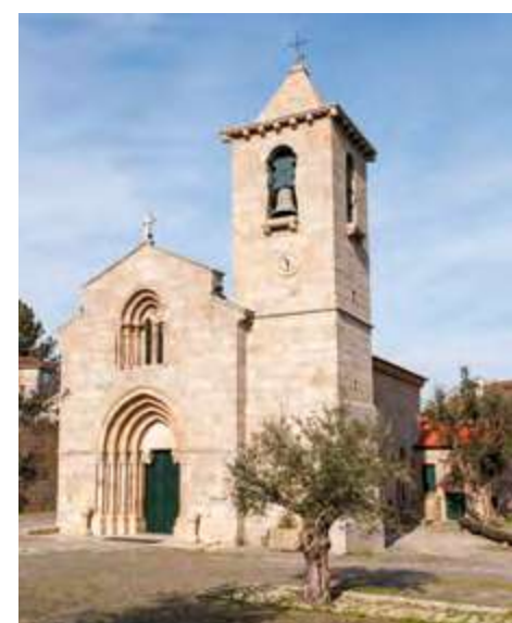
West and south façades and bell tower.
