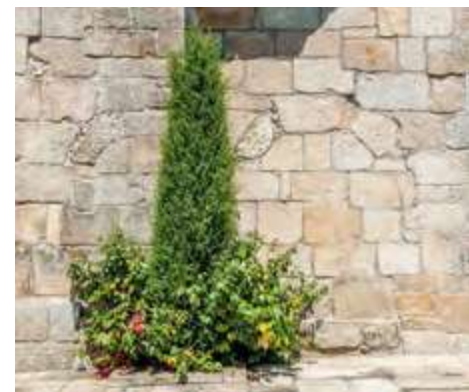
South façade. Nave. Traces of arches.
