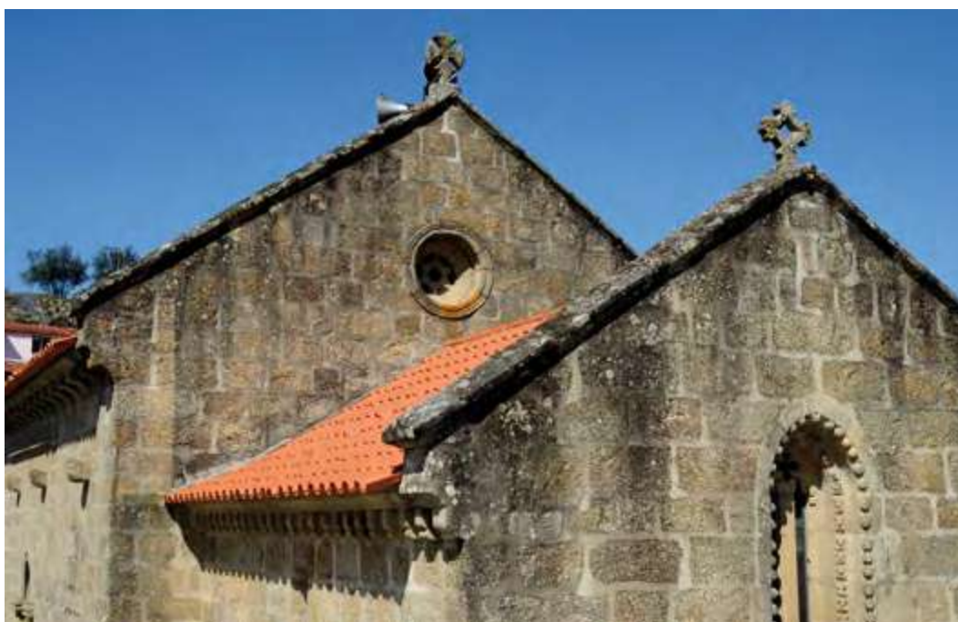
East façade. Oculus and window detail.
