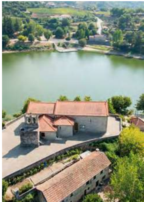
Churches of Sobretâmega and Saint Nicholas. Aerial view.
